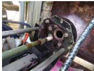
Automated nozzle repair in the field
