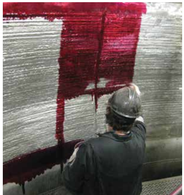
Weld overlay PT inspection
