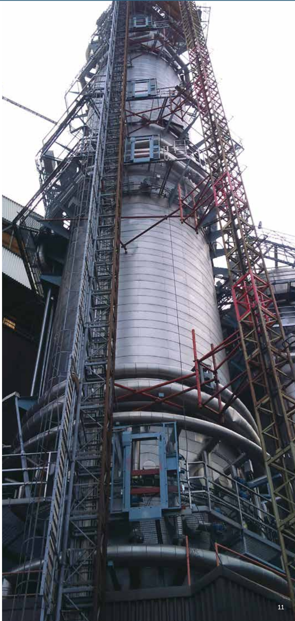
WSI repair on a Digester
