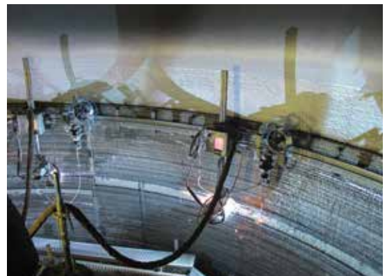
Automated weld overlay using the Unifuse process
