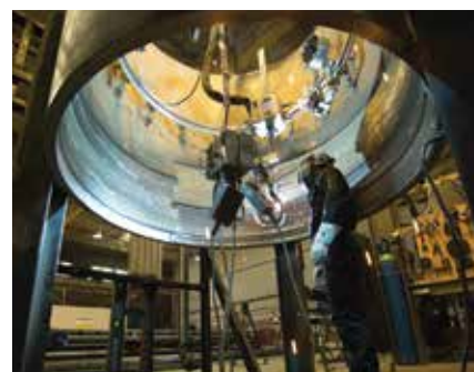
Mock-up for automatic weld overlay
