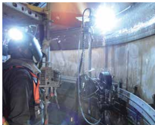
Workforce is fully equipped with necessary safety materials
